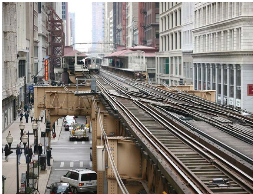
Elevated tracks in the Chicago Loop (US)
