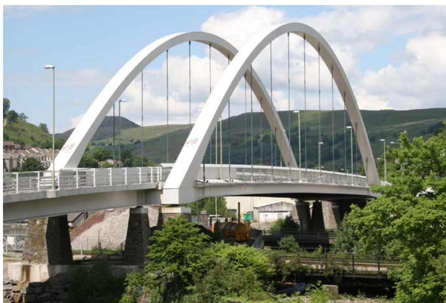
Rheola Bridge, Porth (UK)
